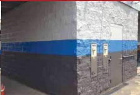
Control Room After
